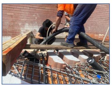
The use of custom shaped glass-fibre reinforced polymer rods meant that the 200 millimetre thick and curved artistic form of the main "shield", using low-strength 25 MPa limestone aggregate concrete, could be inscribed following casting by the artists.<sup>1</sup>
