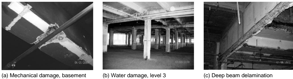
Figure 3. Damage to Beams, 726 Hay St
