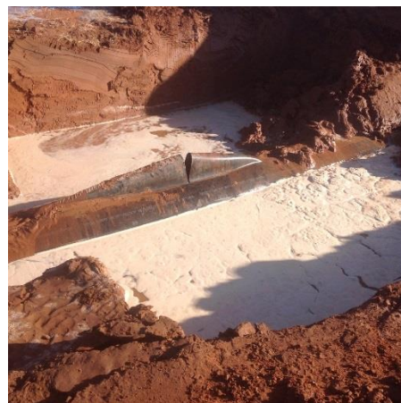
Photograph 1: is a photo of the failed pipe in the trench before dewatering and removal.
