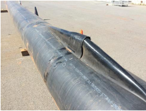
Photograph 2: is a photo of the failed length of pipe after it was transported to Perth for detailed inspection and testing.
