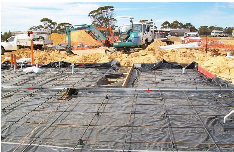
Irrigation points in place prior to slab pour at Merredin Residential College
