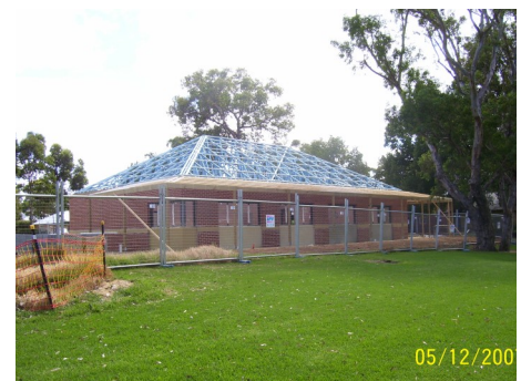
Library nears completion.
