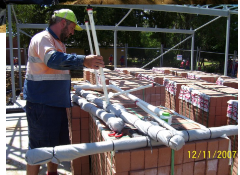
Contractor assembles irrigation system to supply up-hill side of sand blanket.
