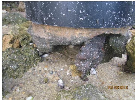
Figure 1. Left: Steel UC Connecting to Steel Framing. Right: Steel UC Below Concrete Encasing.
