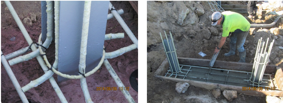
Figure 9. Forming and Pouring of Footings.
