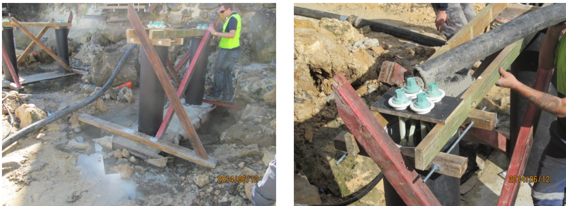
Figure 10. Forming and Pouring of Columns.
