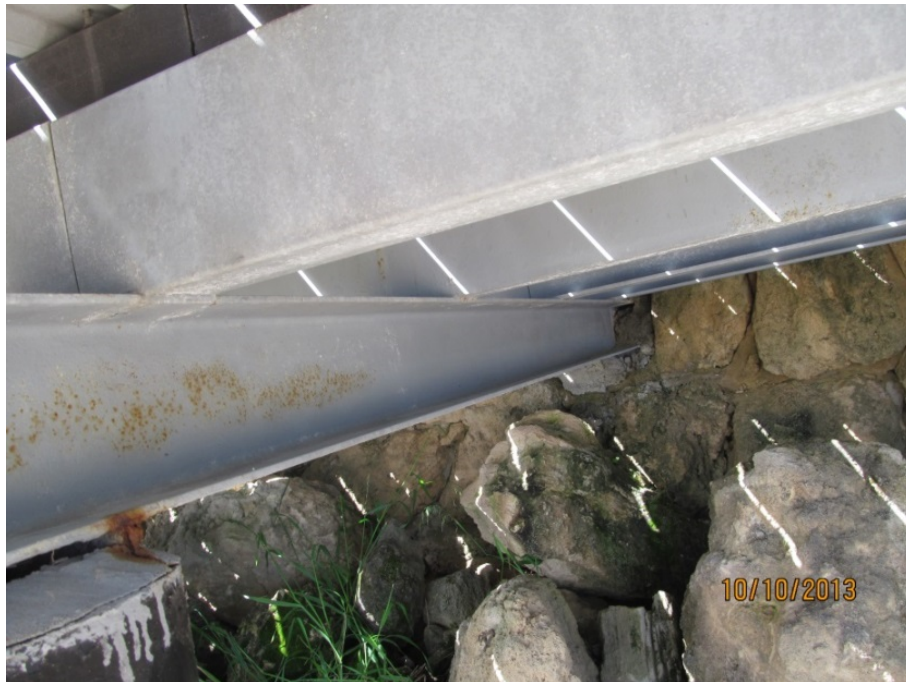
Figure 4. Steel Cross Beam Embedded in Retaining Wall.
