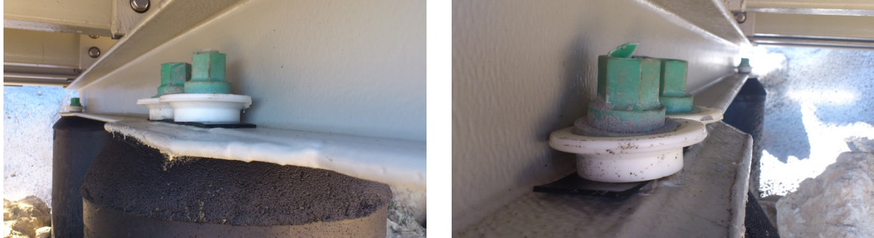
Figure 11. Column and Steel Connection.
