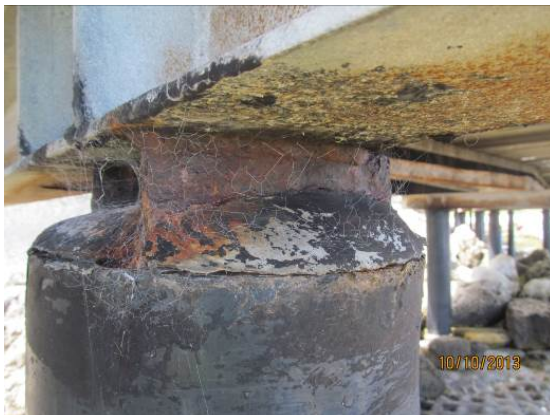
Figure 1. Left: Steel UC Connecting to Steel Framing. Right: Steel UC Below Concrete Encasing.
